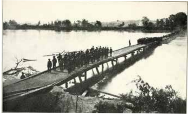
Pontoon bridge across the Big Barren River at Bowling Green, Ky
