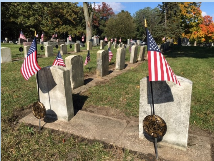
The sod was removed from the bases of gravestones and the stones were cleaned and preserved
