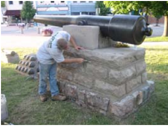
Doug Armstrong tuck-pointing the joints of the cannon base.
